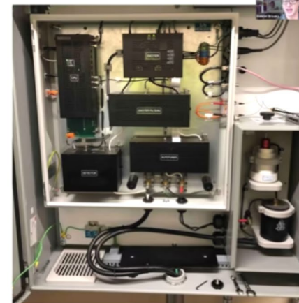
Figure 13. GRS Biomark FS3001 Transceiver with external capacitors – Gabriel Brooks, NOAA
